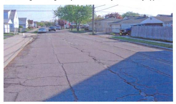
Lafayette St in Lincoln Park was first milled to improve the ride. This is not always necessary. A single chipseal was applied using CM-90 asphalt and 29a slag aggregate in May of 2008.
