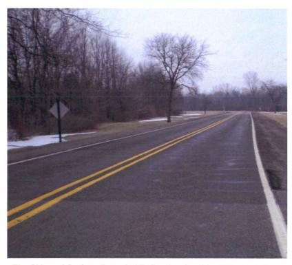
The Chipseal Surface Retarded Reflective Cracking 5 Years Later, As Shown Above, Picture Taken: February 2008
