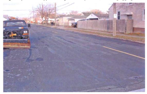
The finished surface after the chip and micro slurry application in December 2008. This surface has extended the life of many such pavements for 6-8 years for one half the cost of mill and overlay prices.
