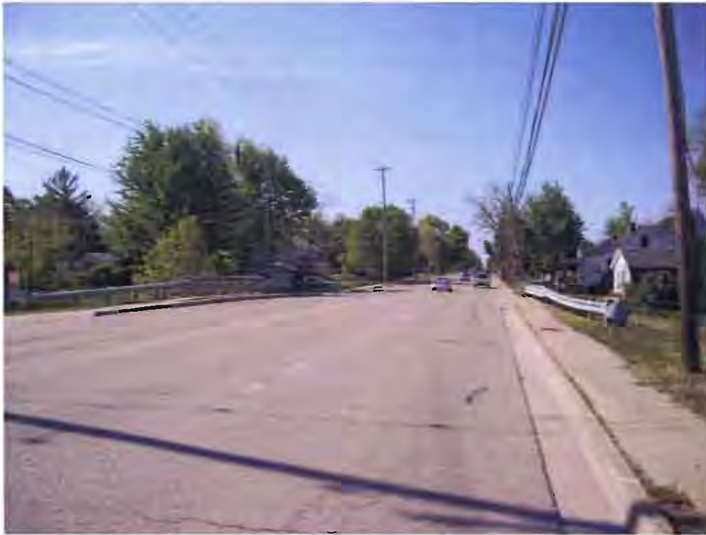
Looking South across Morrish Road Bridge
