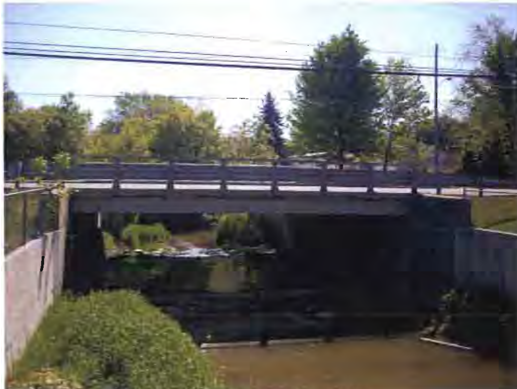
West Side of Morrish Road Bridge
