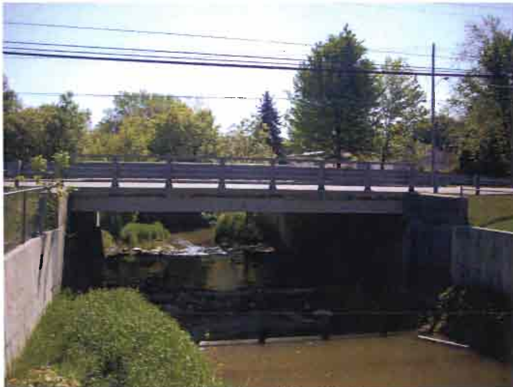
West Side of Morrish Road Bridge
