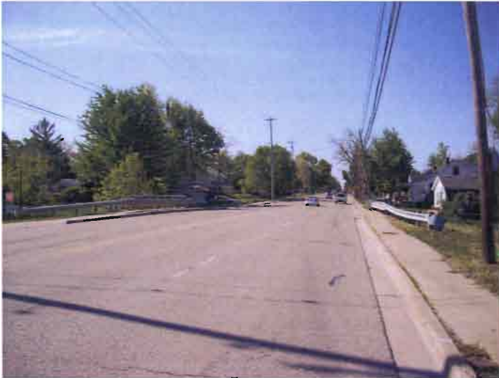
Looking South across Morrish Road Bridge
