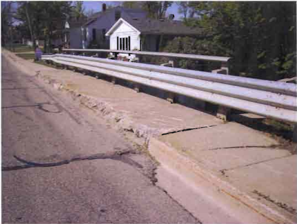
Deterioration of Curb/Sidewalk
