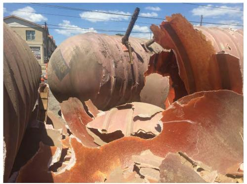
Photograph 11: View of removed gasoline USTs being dismantled.
