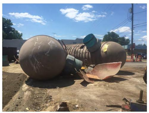
Photograph 10: View of removed gasoline USTs being dismantled.
