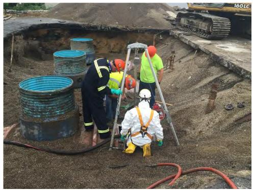
Photograph 9: YECI entering gasoline UST for cleaning.
