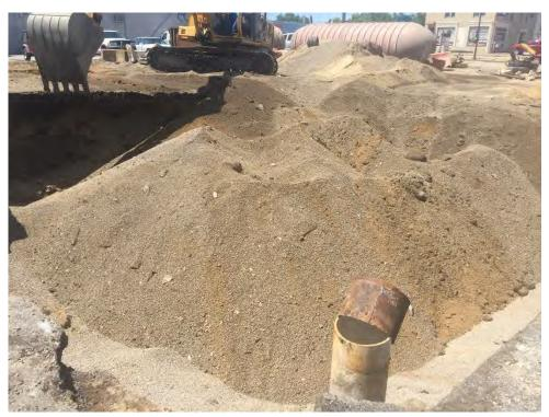
Photograph 12: View of gasoline UST cavity backfill in progress.
