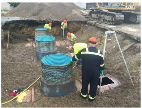
Photograph 8: YECI in the process of cutting the gasoline USTs.
