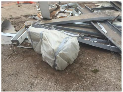
Photograph 5: View of suspected asbestos-containing chimney liner, wrapped in plastic.
