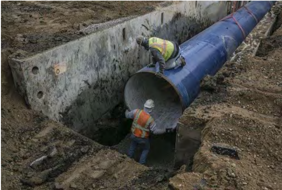
A construction crew works on laying pipe for the Karegnondi Water Authority pipeline along Norway Lake Road in Lapeer in this 2015 Flint Journal file photo. (Sean Proctor | MLive.com)
