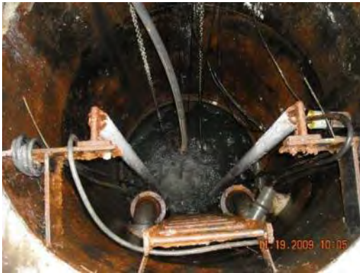
Existing Wetwell with submersible Pumps & Existing Can station Dry Pit
