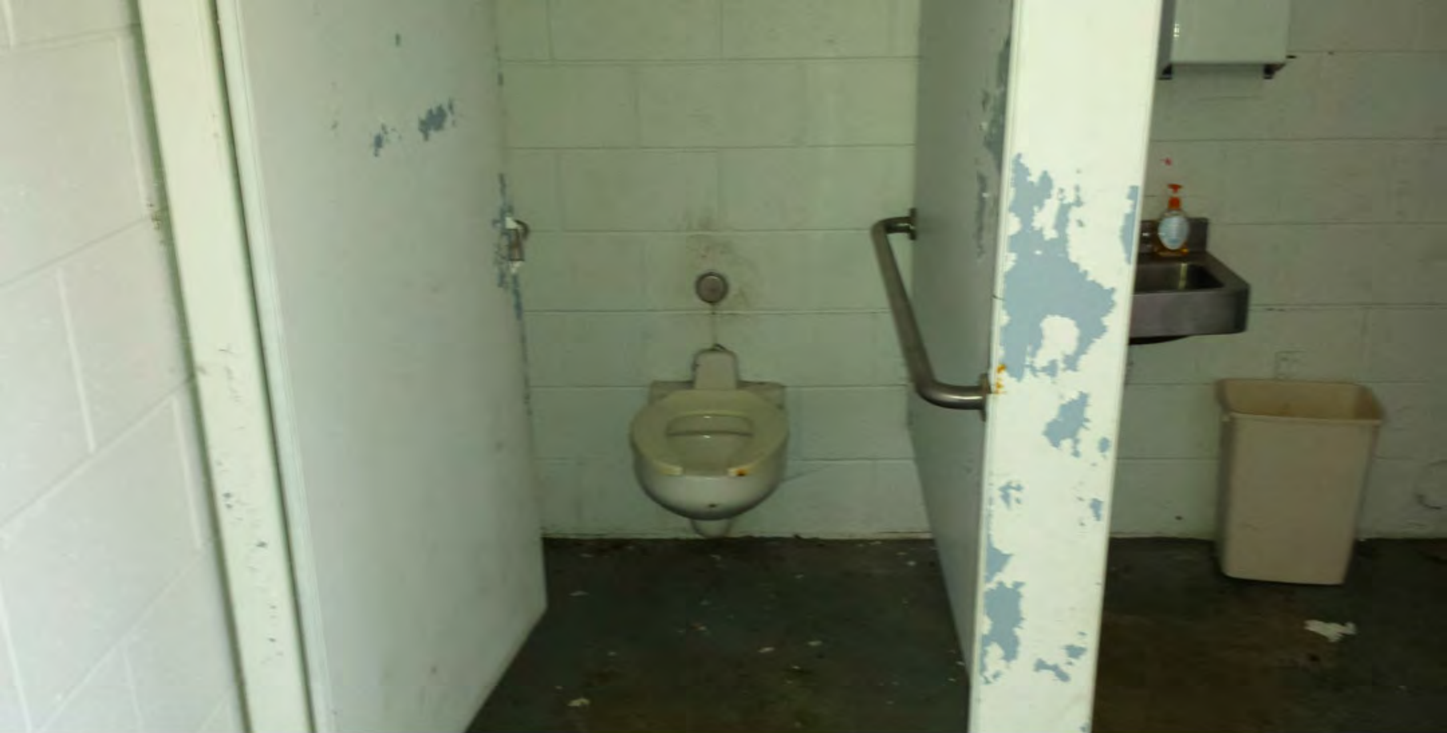
Image 14: Western most stall in women's bathroom, looking east.
