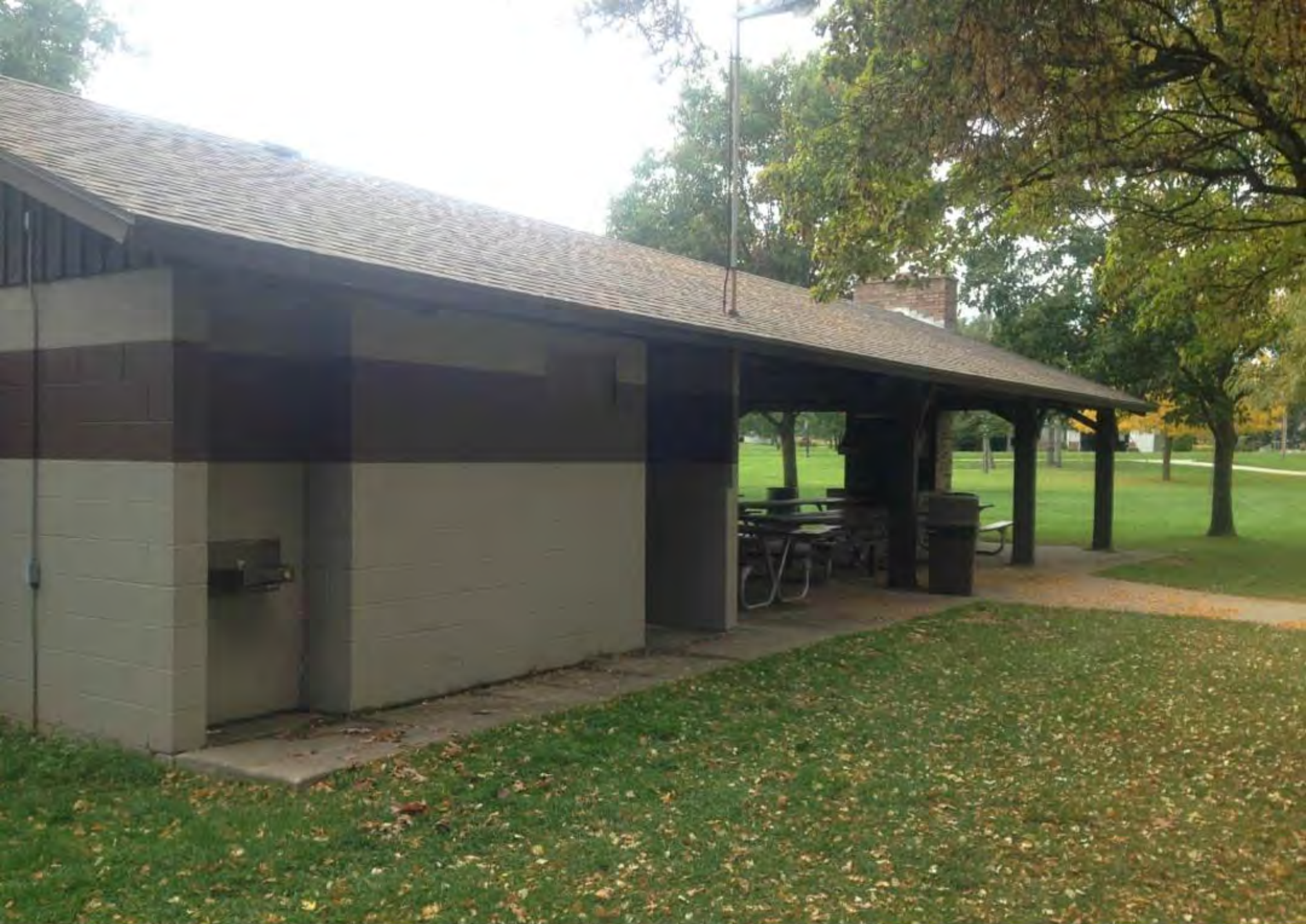
Image 17: Main pavilion and bathrooms, looking southwest.
