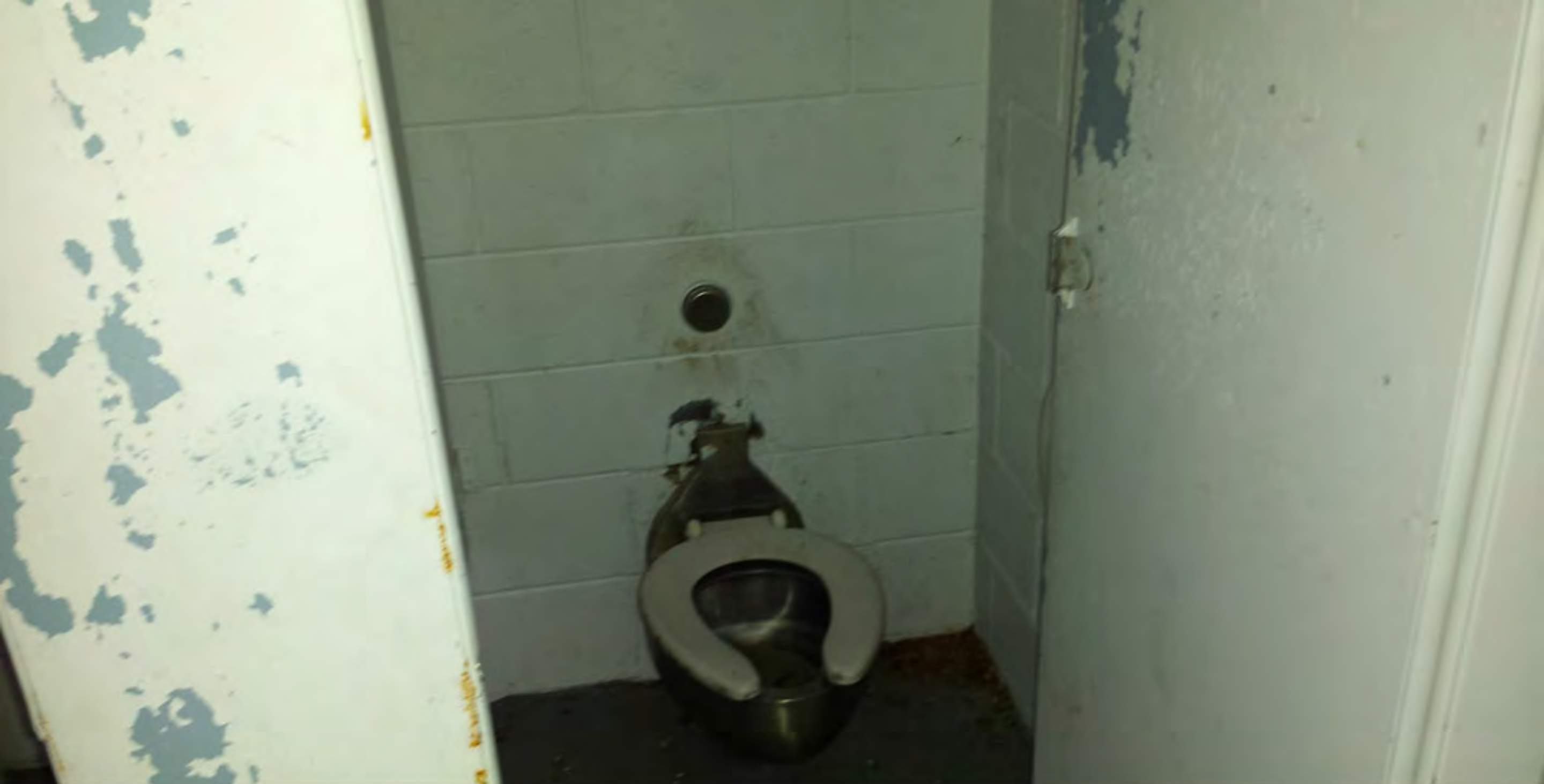
Image 12: Eastern most stall in women's bathroom, looking east.
