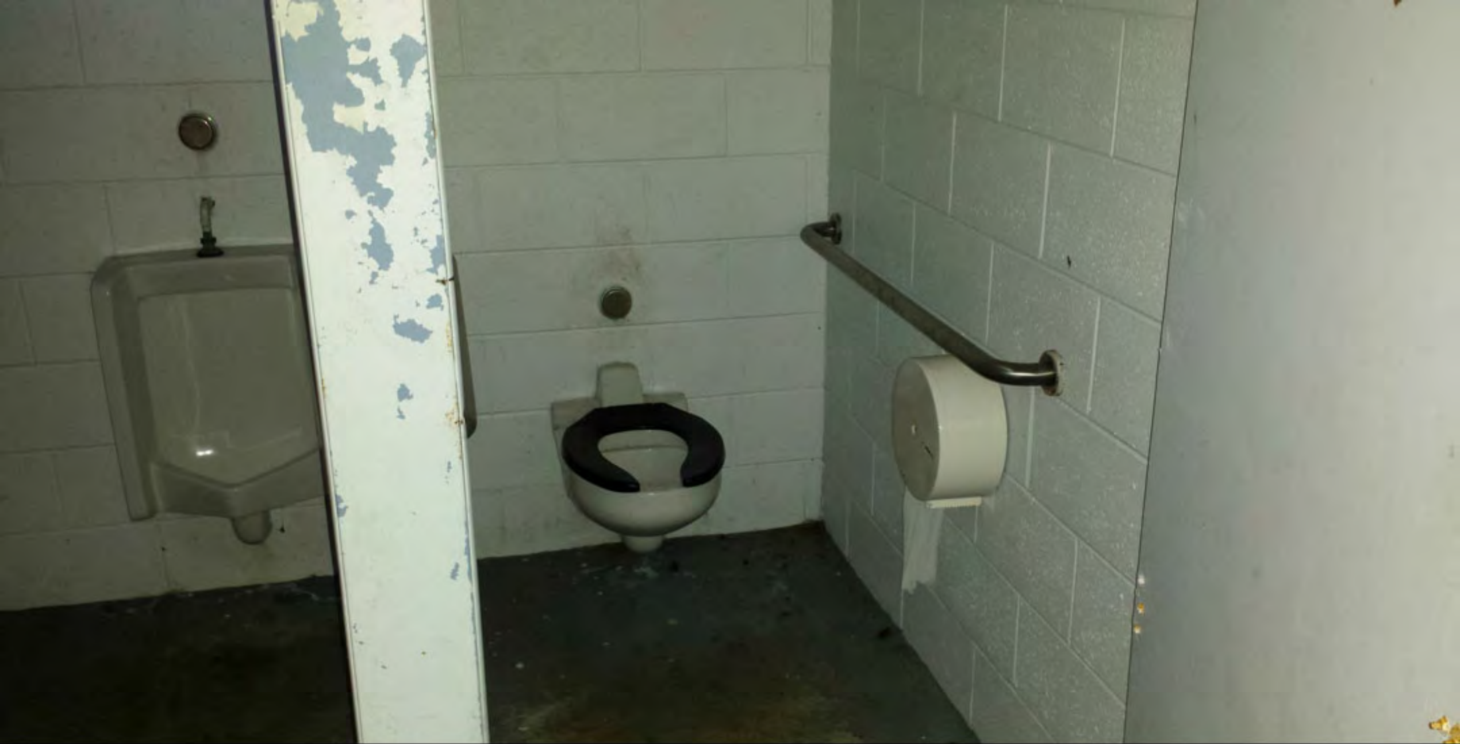
Image 9: Men's stall and urinal, looking east within bathroom.
