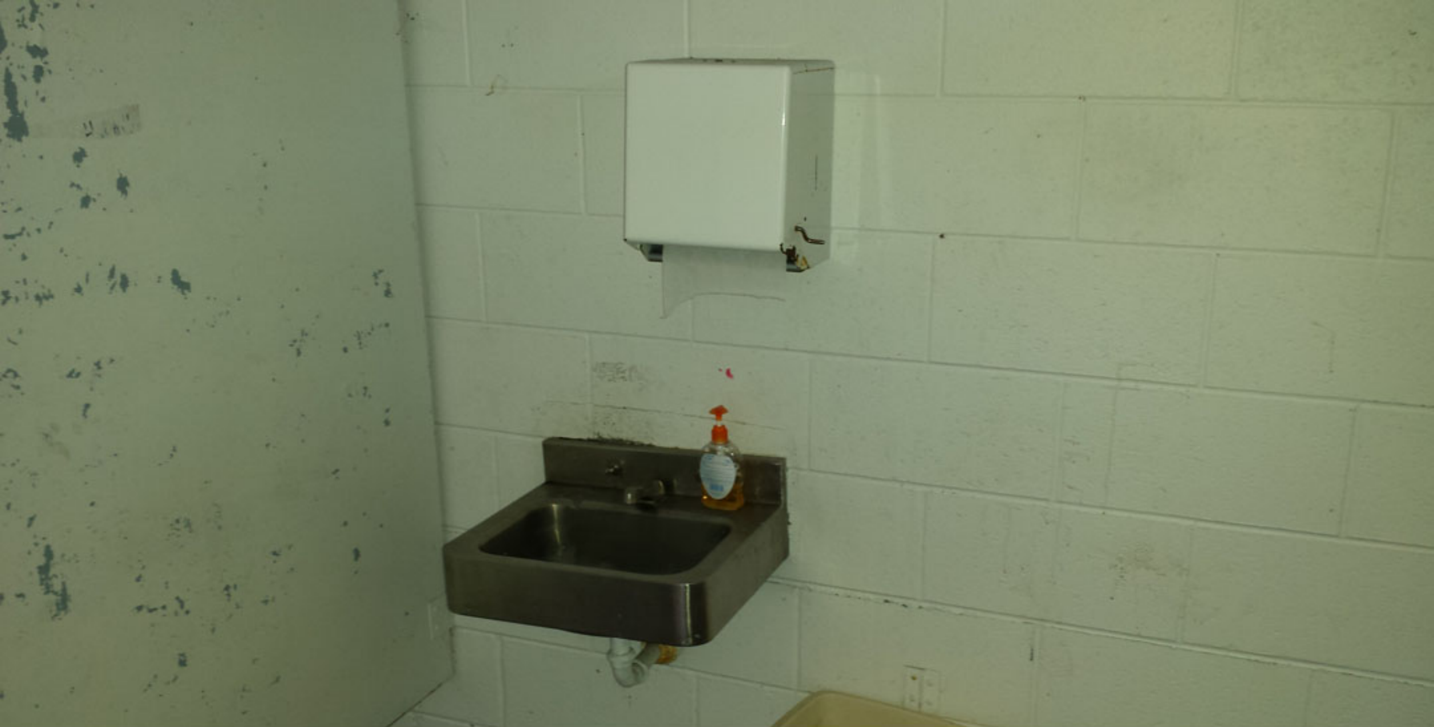
Image 13: Sink, towel dispenser, and western most stall partition in women's bathroom, looking east.
