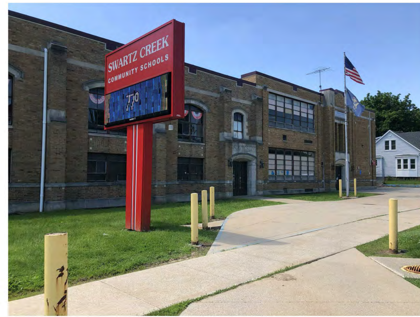
EXISTING NORTH FACADE
