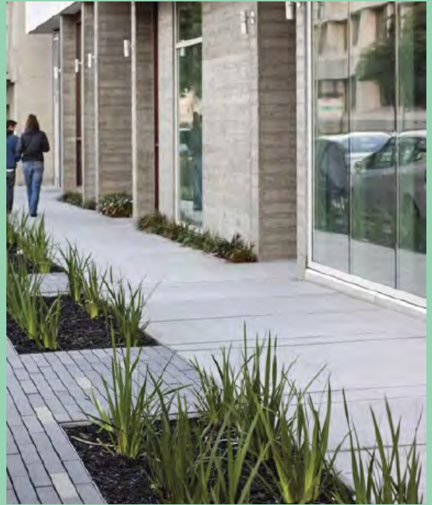
Stormwater areas and porous pavers
