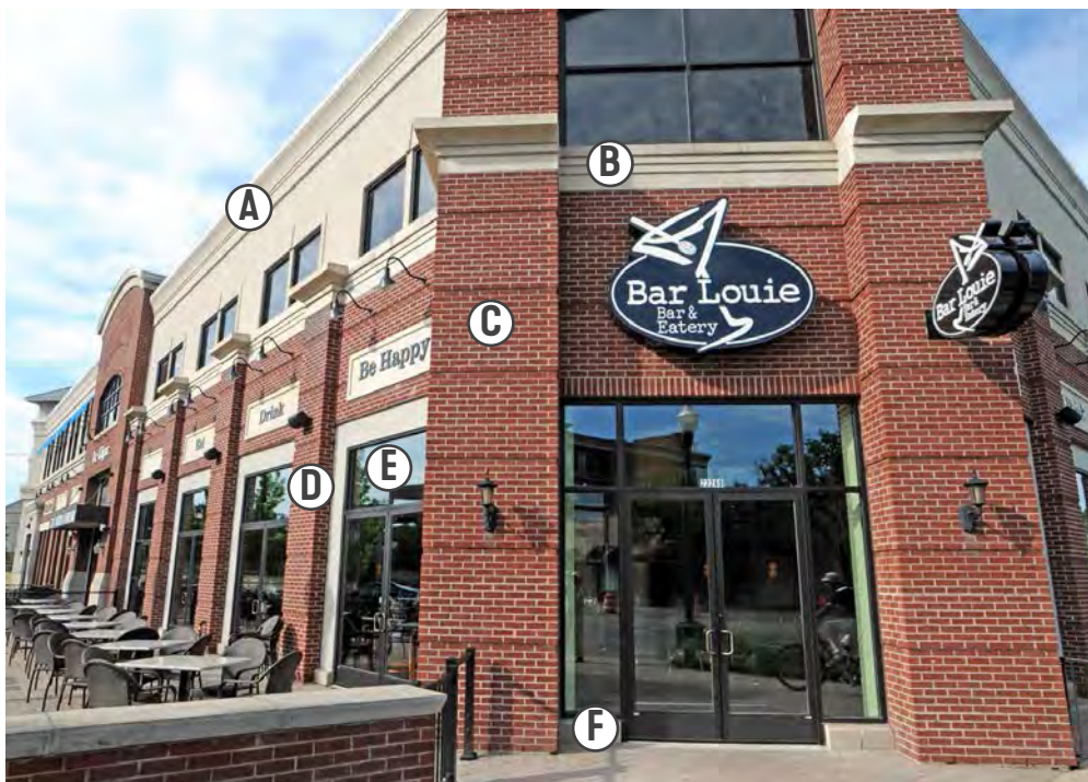
Examples of Architectural Detail:
