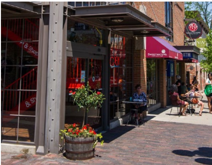
Transitional brick material within the frontage zone
