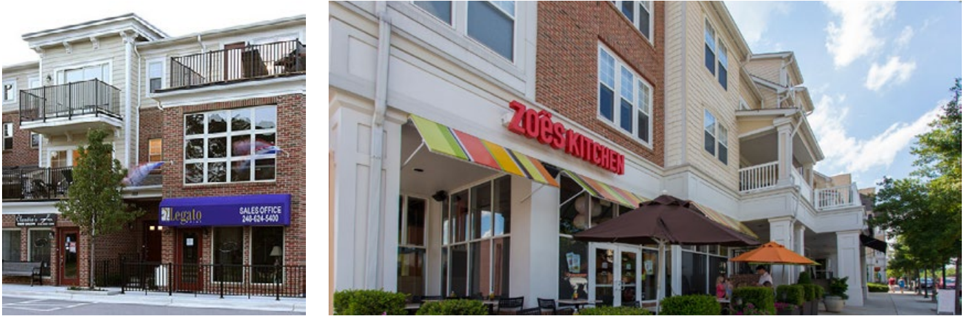
Upper floors are divided into a set of vertical bays through shifts in plane and accompanying material changes.
