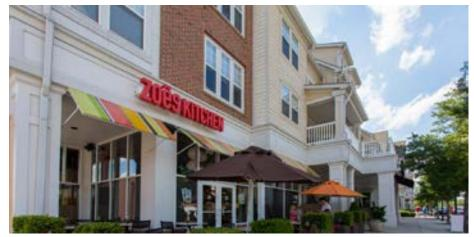
Upper floors are divided into a set of vertical bays through shifts in plane and accompanying material changes.
