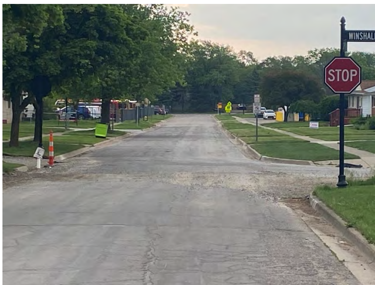
Cappy Lane @ Winshall Drive looking East.
