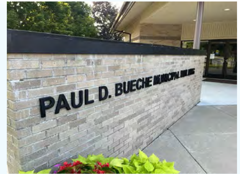
Existing sign and wall
