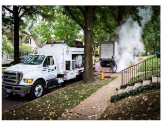
Boiler truck operation during curing of CIPP liner
