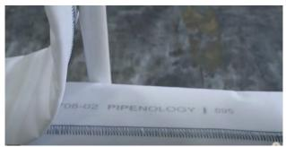
Every Pipenology CIPP liner is stamped with footage markings and an identification number for tracking purposes.
