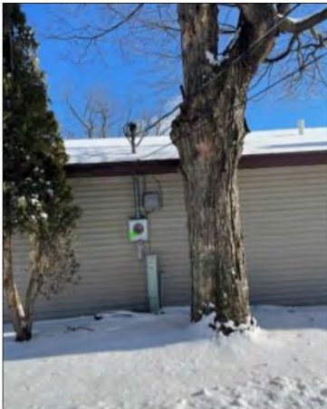
Approved overhead service, meter set only.
