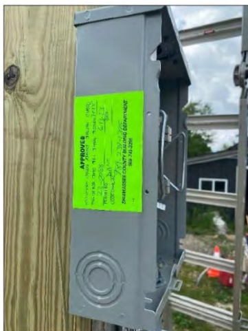
Meter socket inspection sticker.
