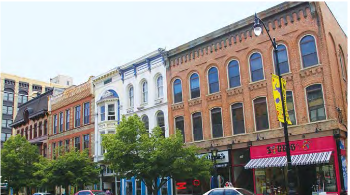
Repetition and order create a harmonious, balanced upper floor design on this building. Materials create accent and detail within a consistent palette.
