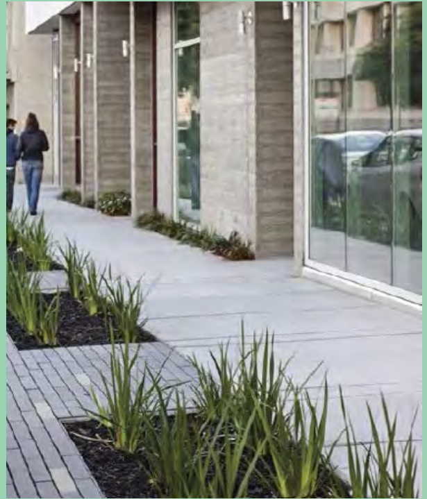
Stormwater areas and porous pavers
