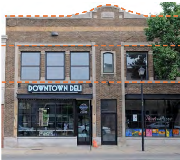
Expression lines create a vertical articulation of base, middle, and top of a façade
