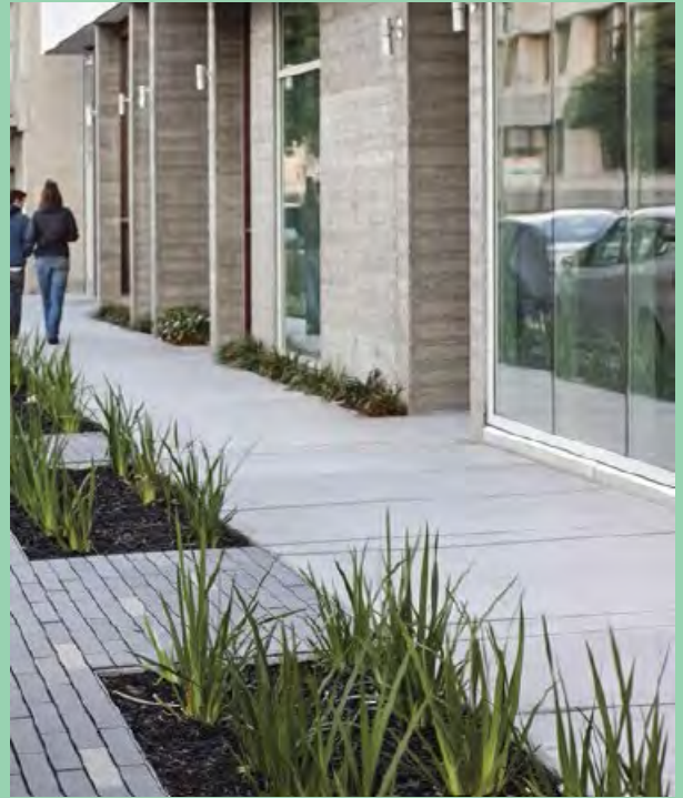
Stormwater areas and porous pavers
