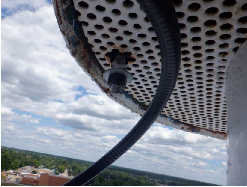
PHOTO #3: Stud extension
